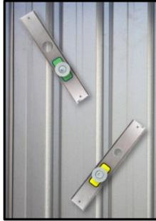
**Step 3.** Screw the bridge bar into the upper flute of the metal deck using screws in the outermost holes, ensuring the Bang-It+ is sticking through the hole in the steel deck.
